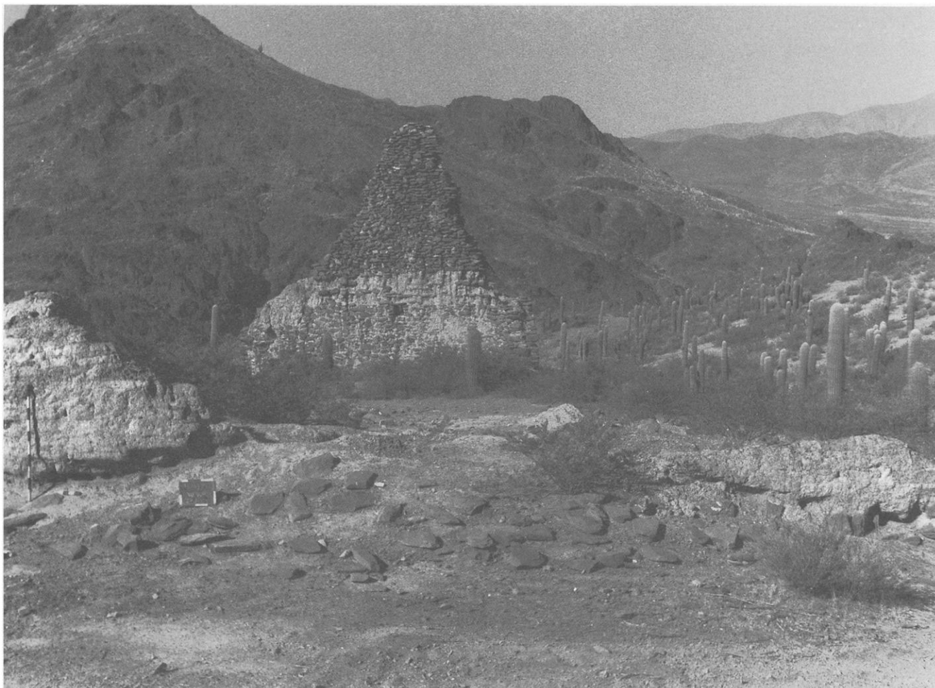
Figure 10. Large kallanka, or gabled hall, bordering the north side of the main plaza at Potrero de Payogasta. End walls were built of stone, adobe and plaster, whereas lateral walls were adobe only; the structure measures about 17 m long \times 8 m wide with one wall preserved to a height of 5 m; view looking east.
